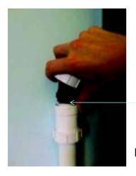
Locate elbow over inner connection and tighten nut.
