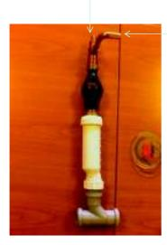
Blow off from Heating expansion vessel
