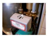
Position far side In this central heating position the spring is powered.
