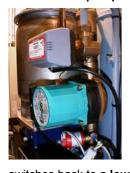
The boiler pump transports the system water through the primary heat exchanger and either system or if applicable internal HWS-tank / or the external cylinder.
