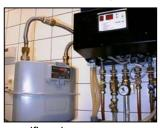
the gas consumption. If the ascertained deviation in load is no more than 15% of the nominal value, the flue gases can be sufficiently exhausted and there is no clogging. At the end of the check, reset the central heating capacity "P" in the menu to its customer-
