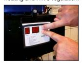
The chimney sweeper function is activated by simultaneously pressing the "+ and the – buttons" of the display in for longer than 5 seconds.
