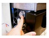
Read the CO<sub>2</sub> value on the analyser. If the value does not correspond with the value in the "CO<sub>2</sub> setting" table, carefully adjust the gas control adjusting screw (2). To do this, temporarily remove the cap (3) with the aid of a Torx screwdriver.
