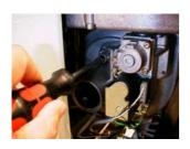
Read the CO<sub>2</sub> value on the analyser. If the value does not correspond with the value in the "CO<sub>2</sub> setting" table, carefully adjust the venturi screw (1). Turn the venturi screw <u>anti-clockwise</u> to increase the CO<sub>2</sub> value, <u>clockwise</u> to decrease it.
