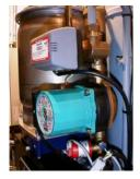
The boiler pump transports the system water through the primary heat exchanger and either system or if applicable internal HWS-tank / or the external cylinder.
