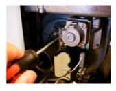
Open the outlet pressure measurement nipple of the gas control
