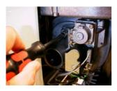
Read the  $CO_2$  value on the analyser. If the value does not correspond with the value in the " $CO_2$  setting" table, carefully adjust the venturi screw (1). Turn the venturi screw <u>anti-clockwise</u> to increase the  $CO_2$  value, <u>clockwise to decrease</u> it.
