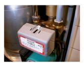
**Position far side** In this central heating position the spring is powered.
