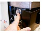
Read the  $CO_2$  value on the analyser. If the value does not correspond with the value in the " $CO_2$  setting" table, carefully adjust the gas control adjusting screw (2). To do this, temporarily remove the cap (3) with the aid of a Torx screwdriver.
