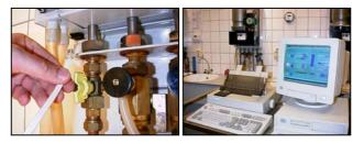
A PC or Laptop can be connected for an extensive diagnosis and display of the functionality.
