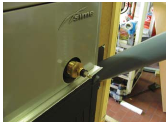
Fig. 28 Safety thermostat
