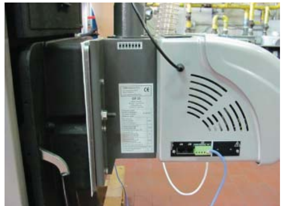
Fig. 26 Fixing of the burner
