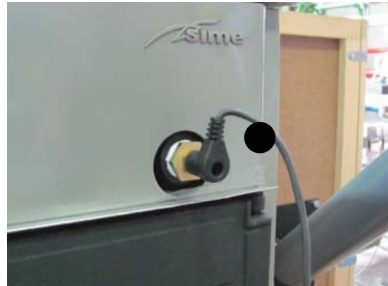
Fig. 34 Safety thermostat connector
