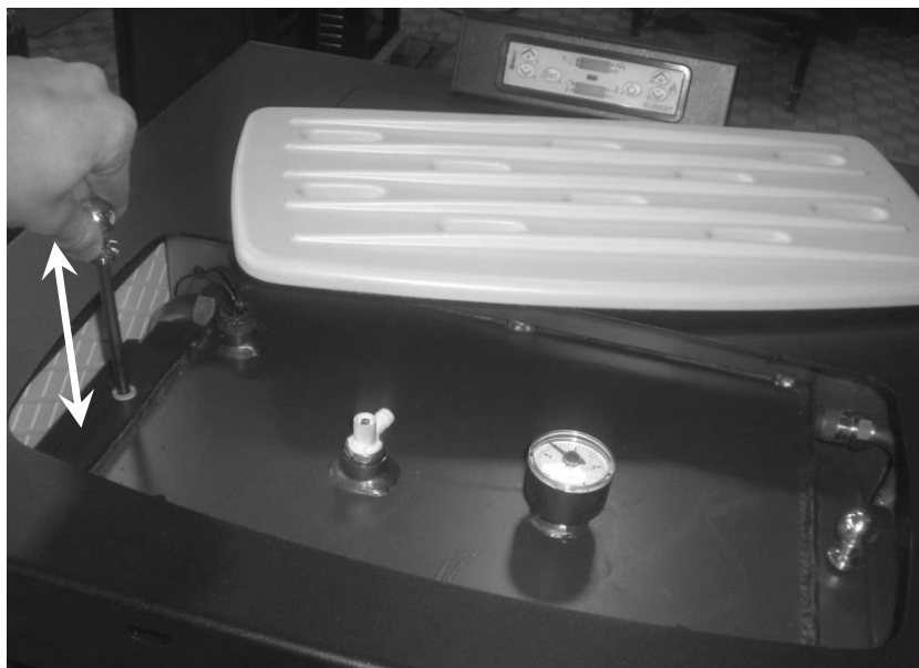
After having removed the majolica top, repeatedly activate the two lateral sticks, to allow cleaning of the flue gas pass.
